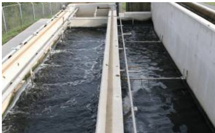
Fig 13.4: Grit and sand removal tank
